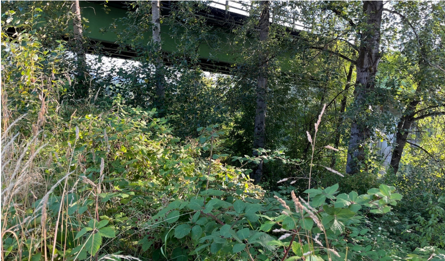
Photo 1. Facing northeast toward E CC St.
